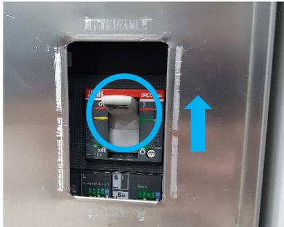
FIGURE 49: MAIN SWITCH "ON"
