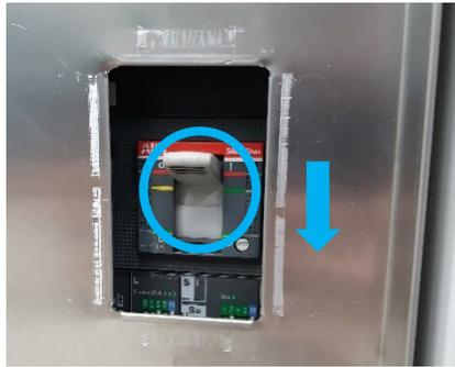
FIGURE 60: MAIN SWITCH "ON"
