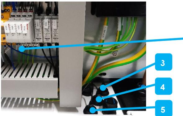
FIGURE 33: INTERNAL COMMUNICATION LINES – PREINSTALLED
