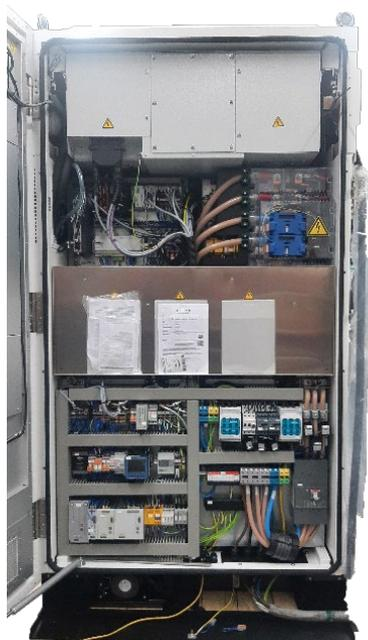
FIGURE 4: VIEW WITH INVERTER SIDE OPEN
