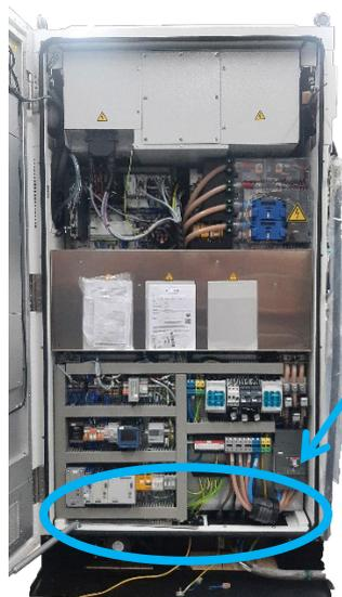
FIGURE 43: CHECKING BASE AREA FOR MOISTURE (INVERTER SIDE)
