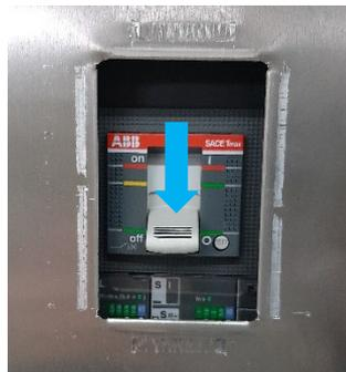
FIGURE 34: MAIN SWITCH IN "OFF" POSITION
