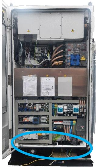
*FIGURE 51: CHECKING BASE AREA FOR MOISTURE
