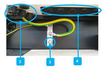
FIGURE 27: EARTH CONNECTION AND CABLE FEED-THROUGHS FROM OUTSIDE
