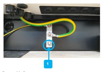
FIGURE 28: CONNECTING THE FOUNDATION EARTH ELECTRODE
