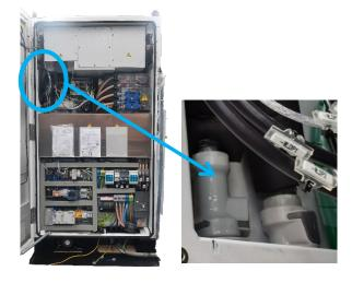
FIGURE 50: CHECKING COOLING HOSES (INVERTER SIDE)
