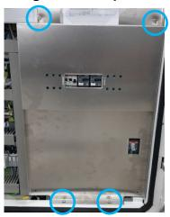
FIGURE 25: ATTACHING COVER PLATE TO MAIN SWITCH
