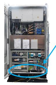
FIGURE 43: CHECKING BASE AREA FOR MOISTURE (INVERTER SIDE)
