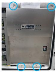
FIGURE 24: DETACHING COVER PLATE FROM MAIN SWITCH
