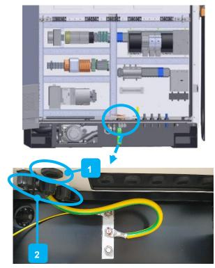
FIGURE 31: POSITION OF CONNECTIONS FOR EXTERNAL COMMUNICATION LINES
