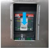
FIGURE 35: SRC4 KEY SWITCH IN "OFF" POSITION
