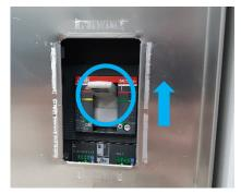
FIGURE 49: MAIN SWITCH "ON"
