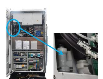
FIGURE 42: CHECKING COOLING HOSES (INVERTER SIDE)
