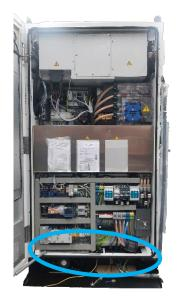
FIGURE 51: CHECKING BASE AREA FOR MOISTURE (INVERTER SIDE)
