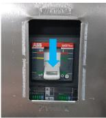
FIGURE 34: MAIN SWITCH IN "OFF" POSITION
