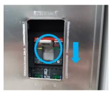
FIGURE 60: MAIN SWITCH "ON"
